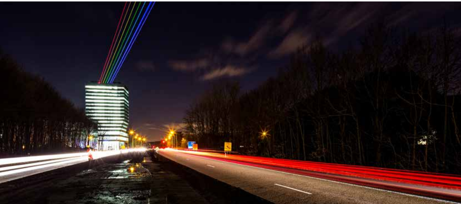
IMEC tower, Heverlee, Belgium Architect: OSAR-BE (Baumschlaeger-Eberle)
