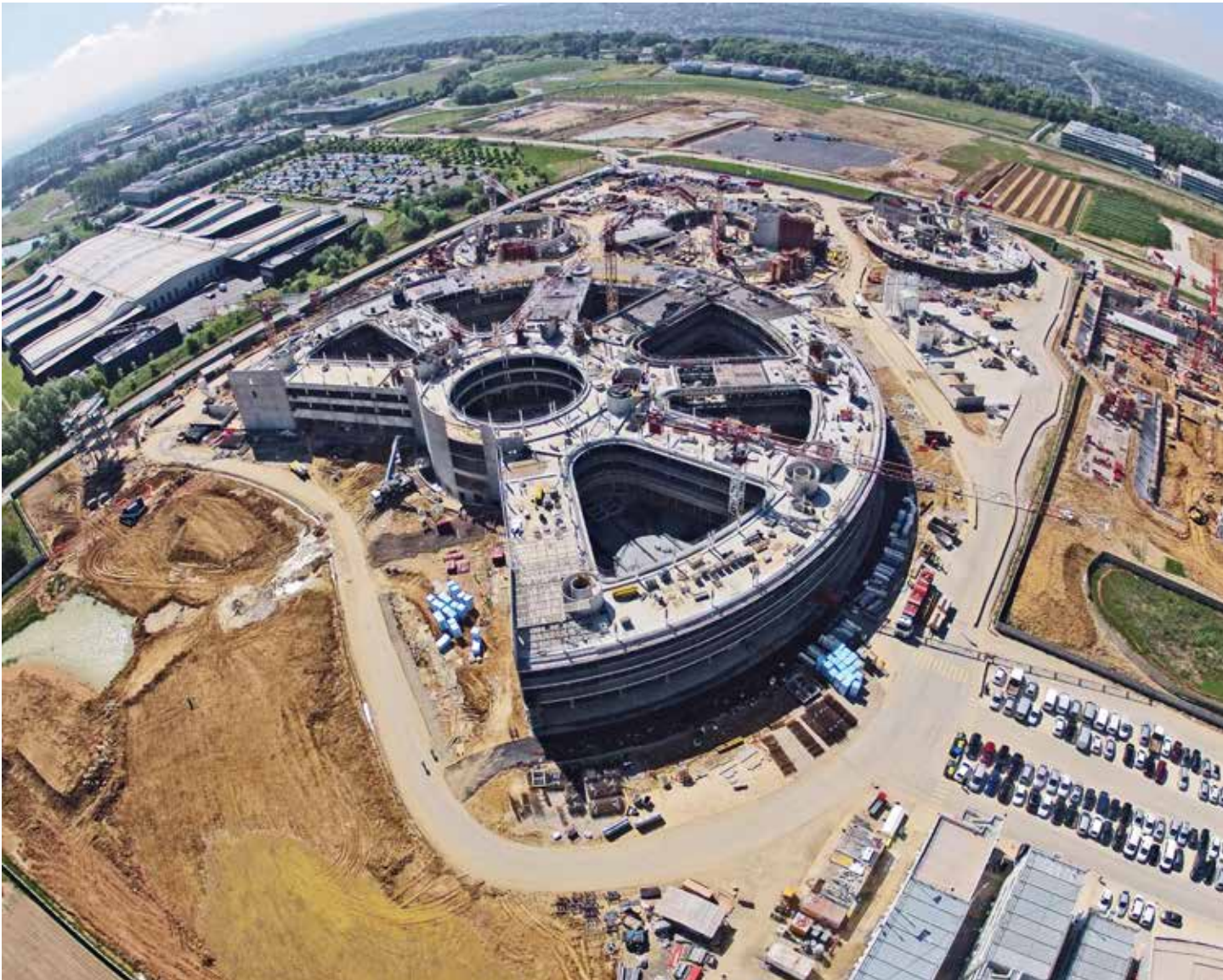
EDF Research & Development centre, Paris-Saclay, France, Architect: Francis Soler
