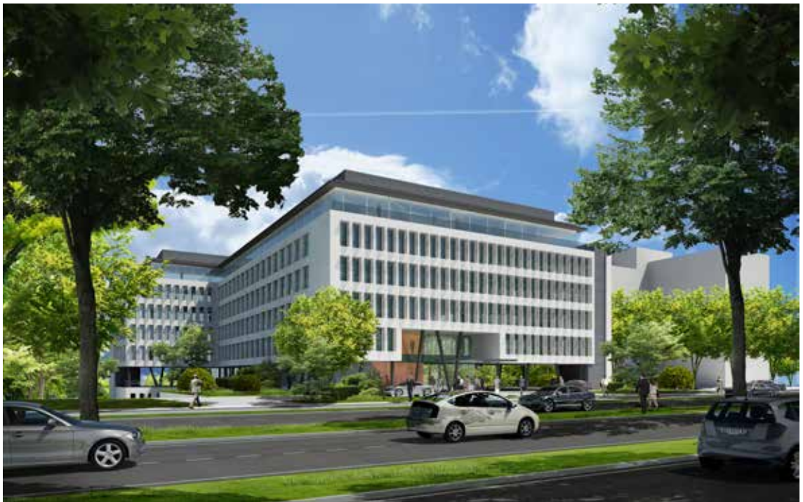
City Gates offices, Senningerberg, GD Luxembourg, Architect: Assar & Perry Weber
