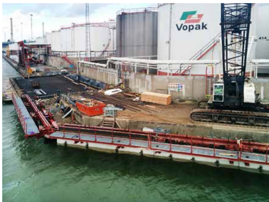
'Vijfde Havendok' (fifth port dock), Antwerp, Belgium
