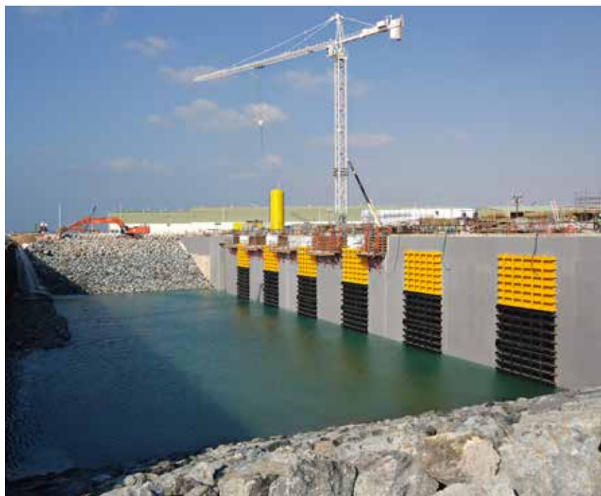
Hamriyah seawater intake, pumping station and outfall channel, Dubai, UAE
