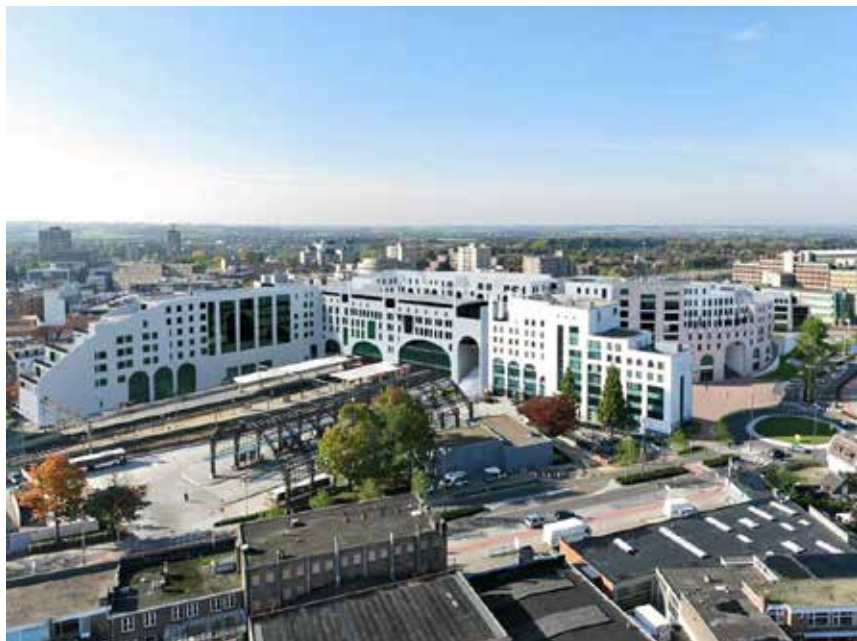
Maankwartier station, Heerlen, The Netherlands Architect: J. Bak, Concept: Michel Huisman
