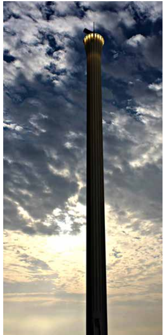
Radar tower 'Neeltje Jans', North Sea, The Netherlands Architect: Paul Wintermans
