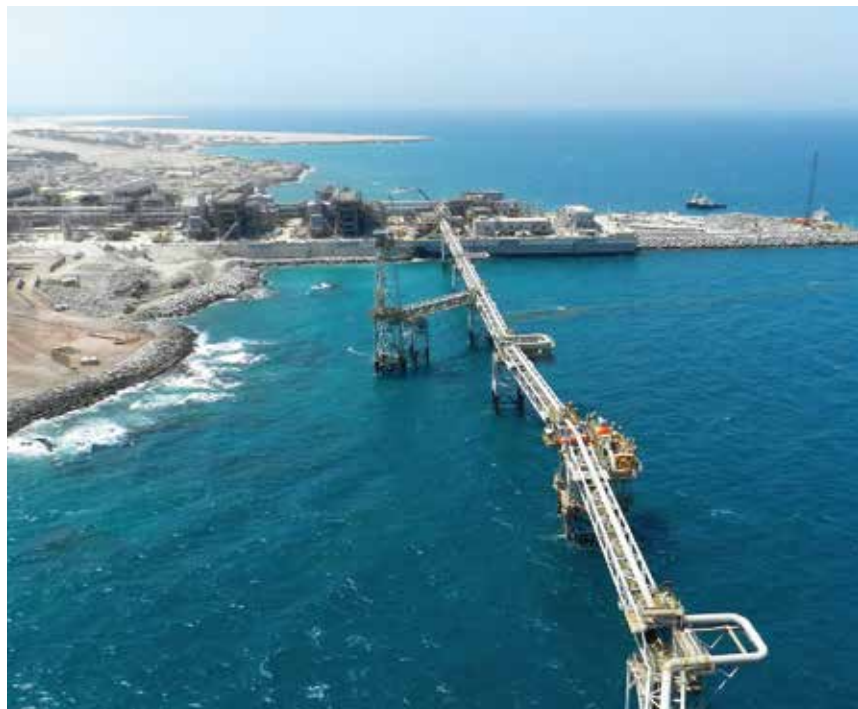
Marine terminal and seawater intake, Das island, Abu Dhabi, UAE
