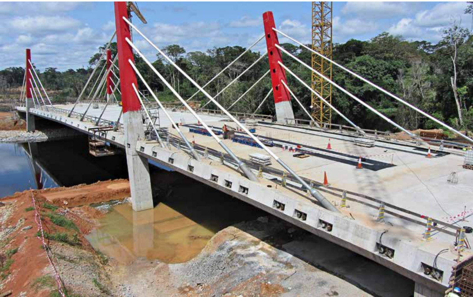
Oyala cable-stayed bridge, Equatorial Guinea
